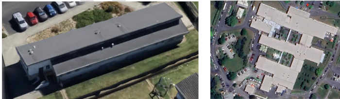
Figure 12: Example of an IL2 Oral Health Centre (dental clinic) generally using NZS 3604 and B2/AS1 (left); and a single storey IL4 Acute Facility, constructed in a mixture of timber framing and structural steelwork (right).
